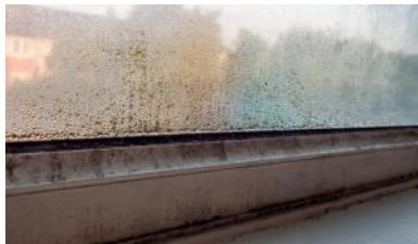
**Condensation:** The most common form of damp caused when warm, moist air comes into contact with cold surfaces like windows or walls. It often leads to **mould growth**, especially in poorly ventilated areas like bathrooms and kitchens.
