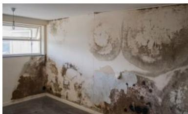
**Penetrating Damp:** Occurs when water enters the building through external defects such as cracked walls, damaged roofs, or faulty window seals. It can appear anywhere on walls or ceilings and often worsens during wet weather.
