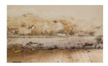
**Rising Damp**: Caused by moisture from the ground moving up through walls due to a failed or missing damp-proof course. It typically affects lower parts of walls and can cause paint to peel and plaster to crumble.
