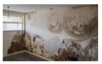
**Penetrating Damp**: Occurs when water enters the building through external defects such as cracked walls, damaged roofs, or faulty window seals. It can appear anywhere on walls or ceilings and often worsens during wet weather.
